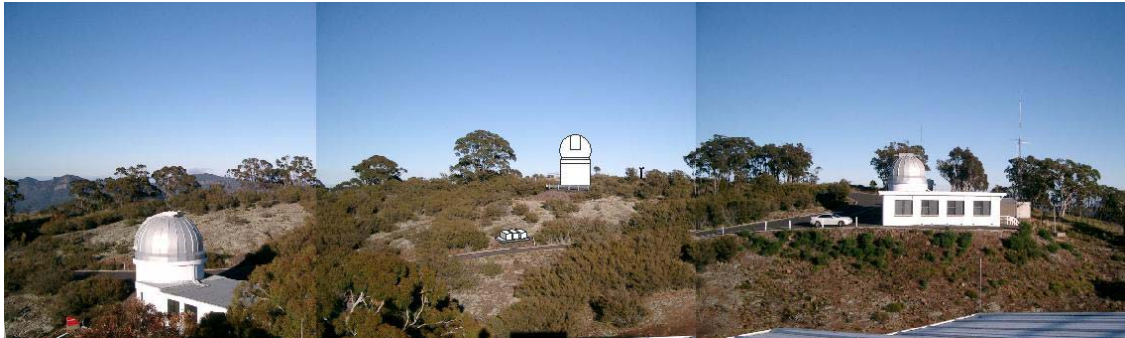
Figure 3: SkyMapper enclosure on the summit, as seen from the roof of the 2.3m Telescope.
