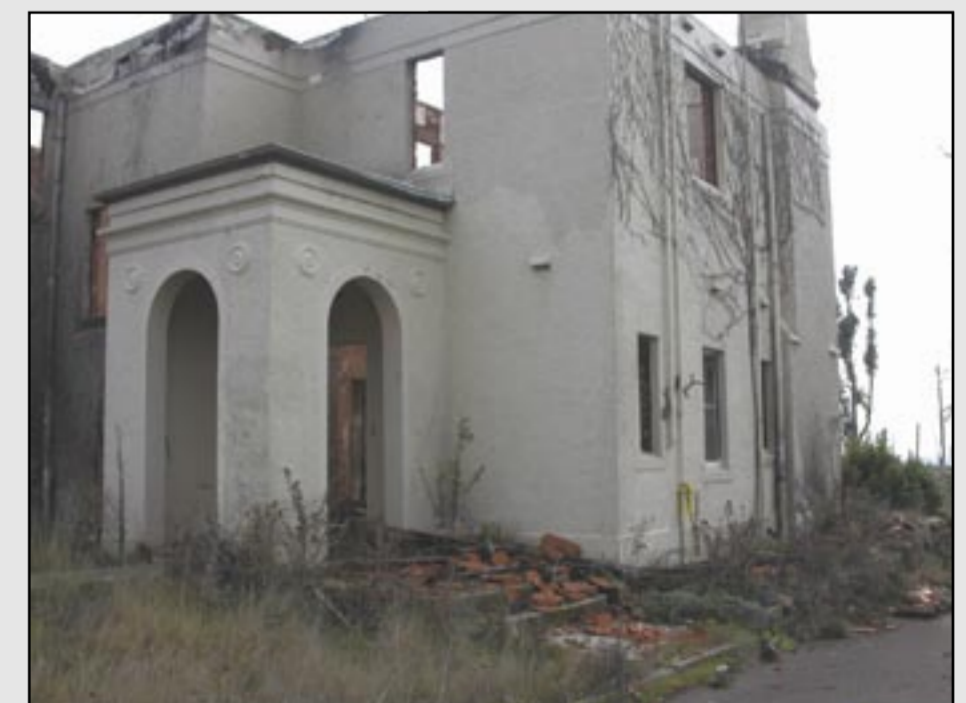
The Director's Residence after the 18 January 2003 firestorm
