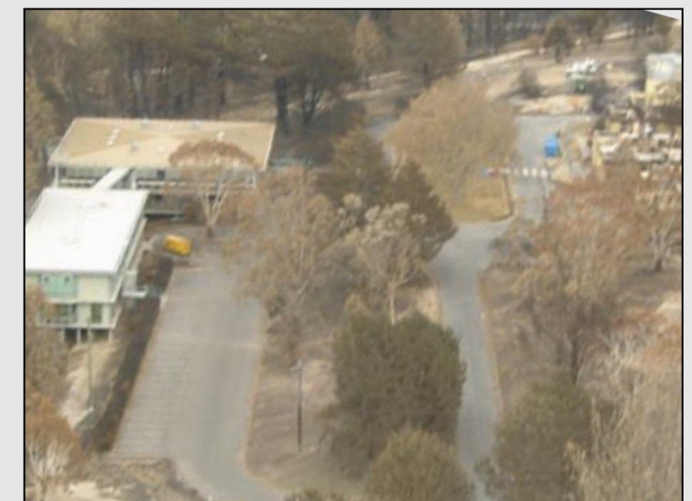
The Woolley & Duffield buildings on 19 January 2003
