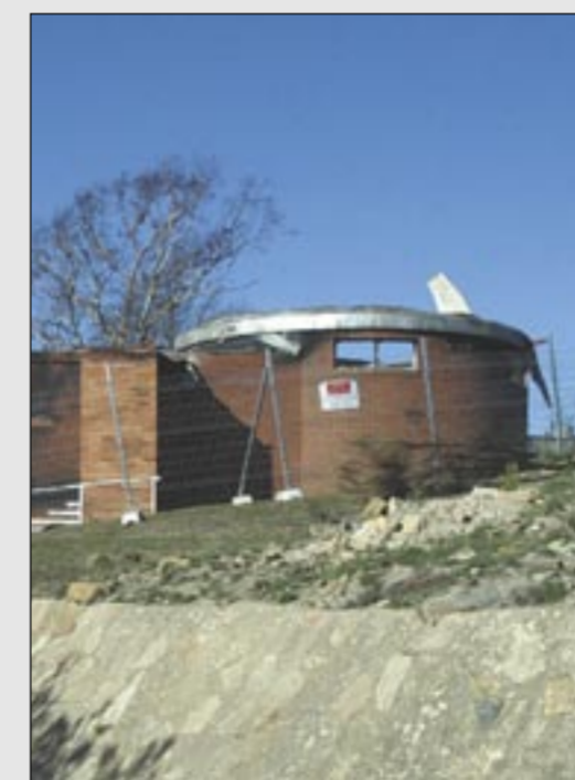
The Uppsala dome after the firestorm
