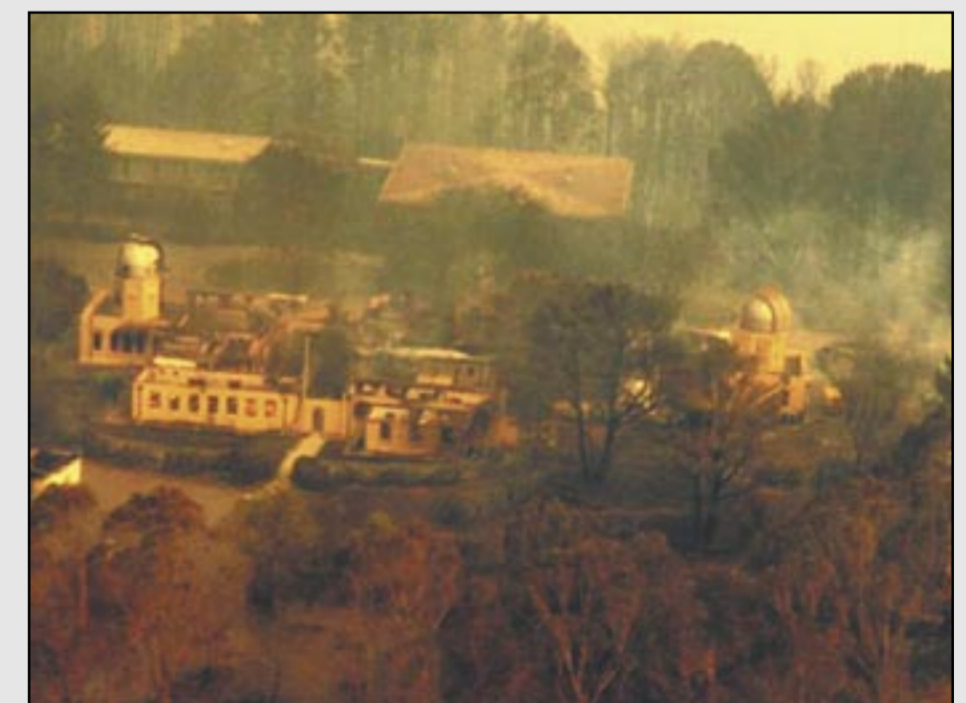
CSO building burning during the firestorm
