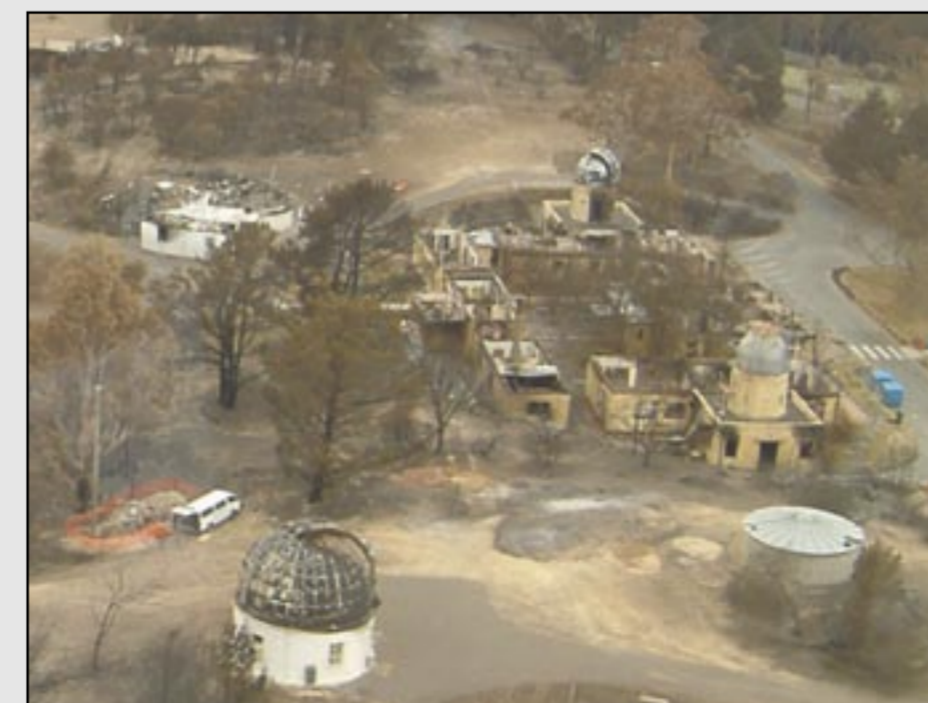
CSO building after the 18 January 2003 firestorm
